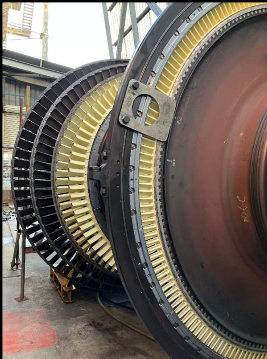
Blades Replaced – HPT, LPT 1, LPT2
