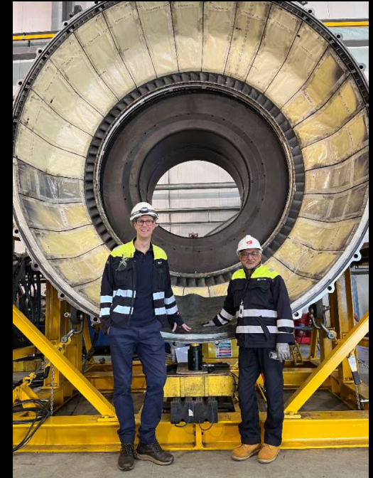
Pre-assembly of Combustor section completed
