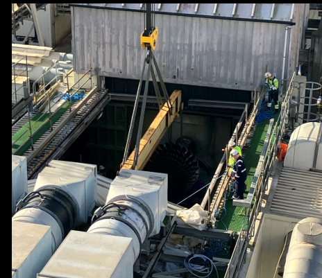
GT Rotor replacement
